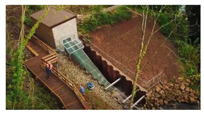
A Micro-Hydro System using the energy produced by the Weir to generate Electrical Power. Havannah Weir will enable the generation of approx. 250,000 kilowatt hours per year, enough to sustain about 60 homes. Operated and maintained by professionally qualified volunteers.
